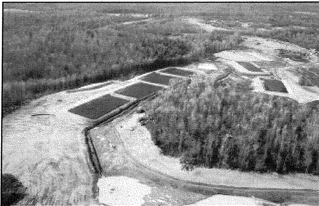
Anna S Mine Treatment System Complex under construction
